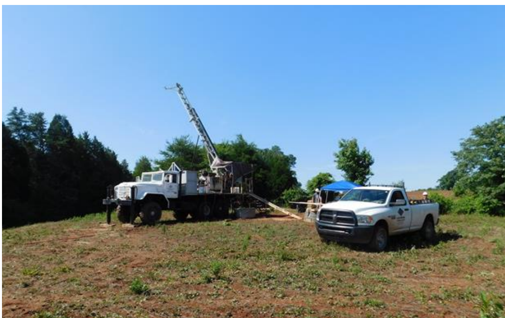
Figure 8: Phase 2 Drill Rig On-Site
